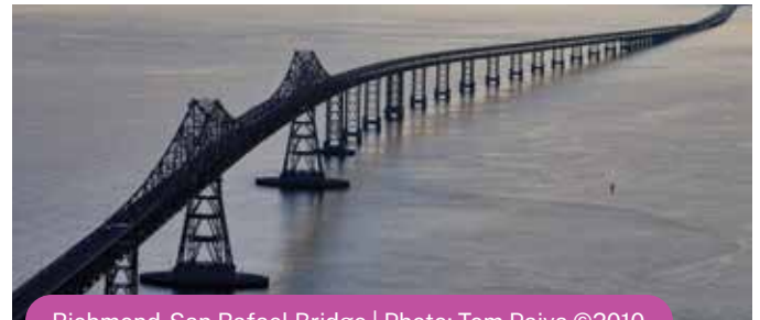
Richmond-San Rafael Bridge | Photo: Tom Paiva ©2010
